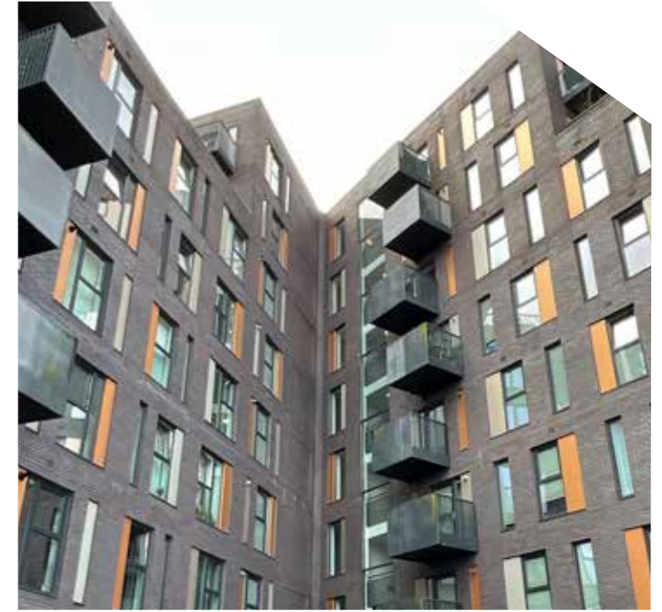
Figure 1 - View of decorative ACM on external walls and balconies
