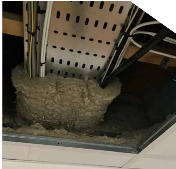
Figure 6 - Picture of compartmentation technique in communal spaces for cable penetrations.
